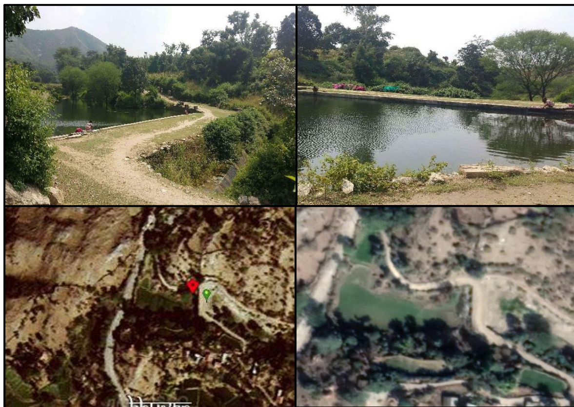
Figure 3-6 Earthen Check Dam, Hathniyawal Village (a) Geotagged Photographs (b) NABARD Bhuvan Portal (c) Google Earth of Vagda Watershed
